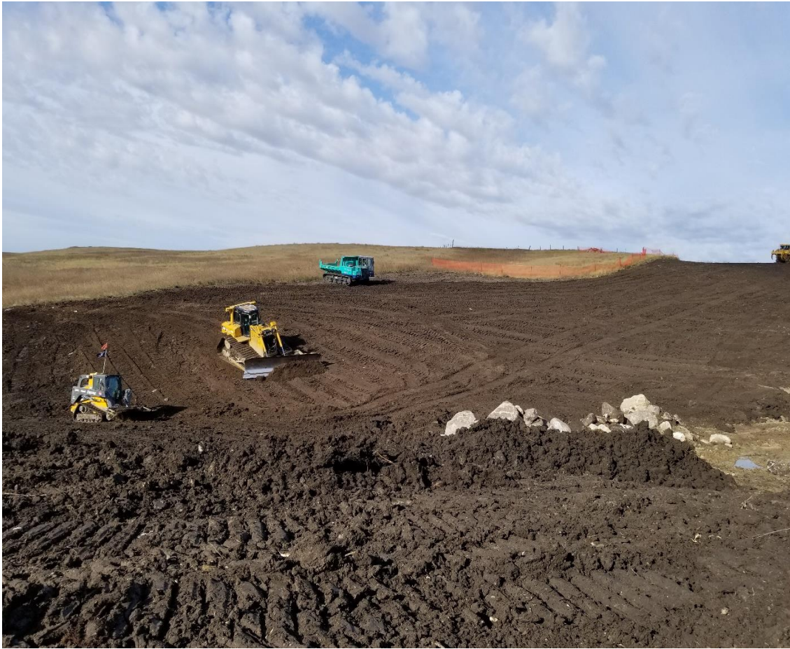
Topsoil being put back at Iskwao creek.
