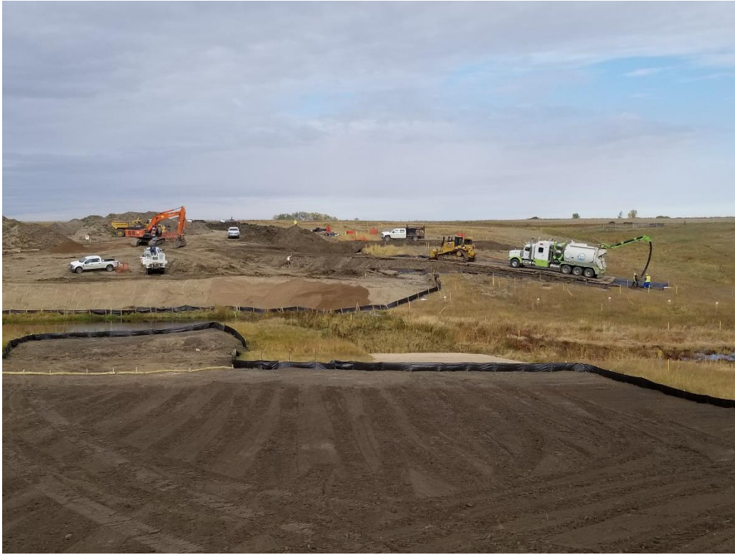
At High Hill Creek the recontouring of slope, crew finishing up the Topsoil.
