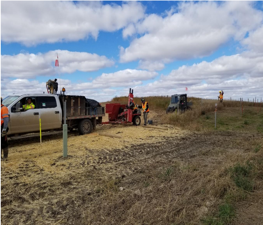
Utility crew installing new fence.
